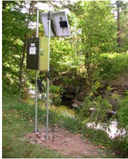
Station along Little Mehoopany Creek, Wyoming County, Pa.
