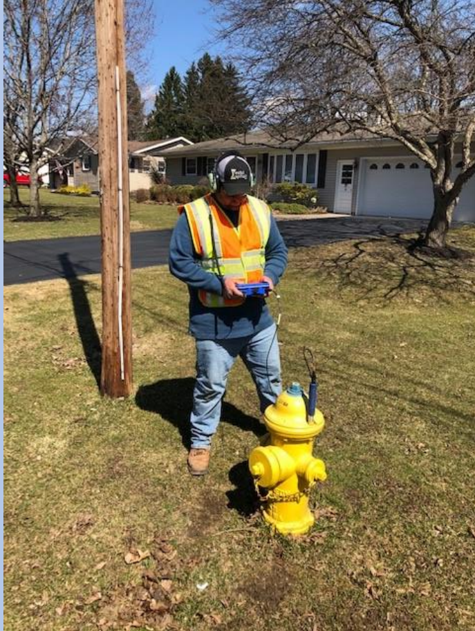
Water operator listens on a hydrant to find a Underground leak
