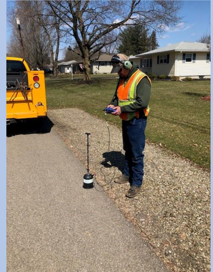
Water operator listens to the ground mic to pin point the underground leak
